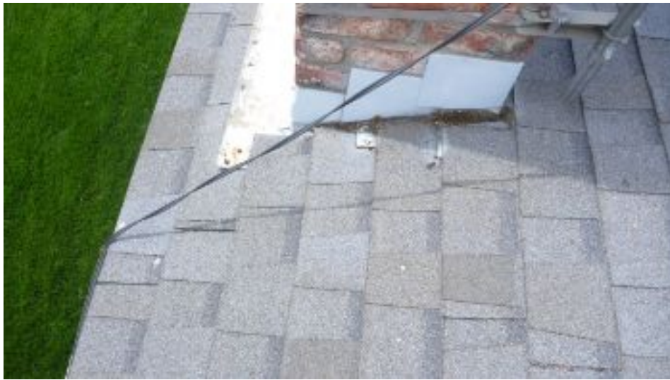
Chimney flashing
